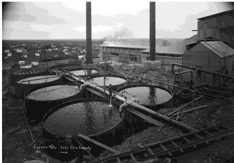
**Figure 5:** Plant and cyanide vats Lake View Consols mine ca. 1896. Note worker inspecting vats (centre). Photo by J.J. Dwyer. Courtesy: State Library of Western Australia.
